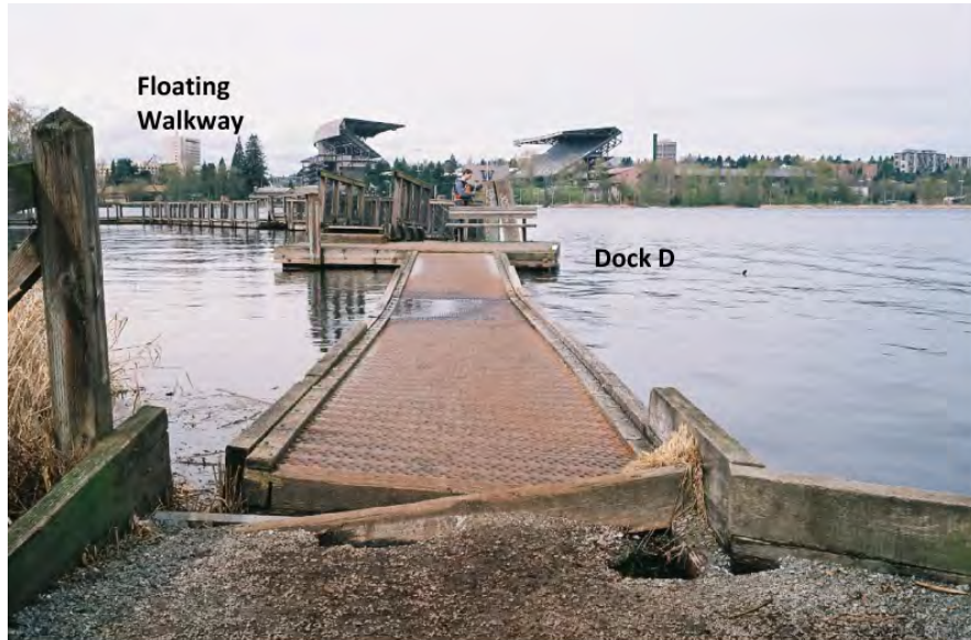
PHOTO No. 2: Dock D, Looking Northwest - Note the Floating Walkway and Dock D in the background. Also note the misalignment of the approach structure and the shoreward erosion.
