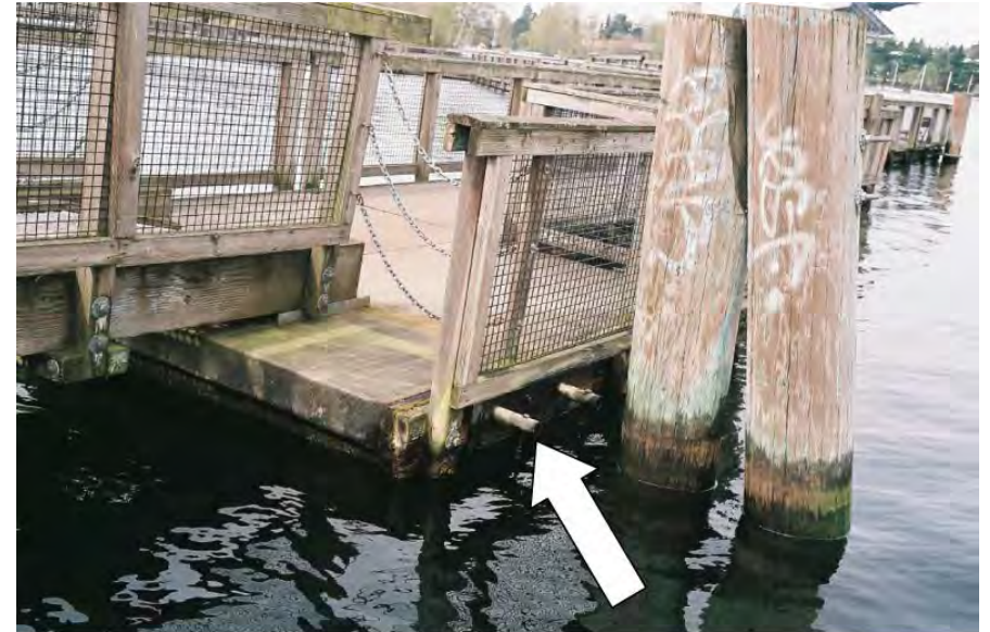
PHOTO No. 7: Walkway, Float Anchor Piles No. 16 and 16 Batter - Note the float anchor hoop is not aligned with the piles and has been cut off. Also note the pontoons are floating unevenly due to the weight of the interconnecting ramp.
